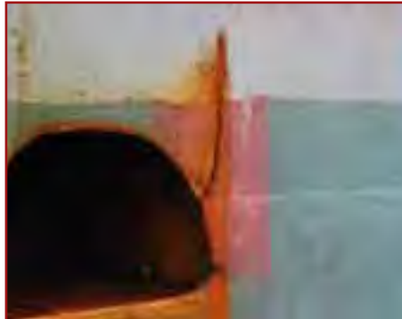
Structural issues, while becoming less common, are still found
