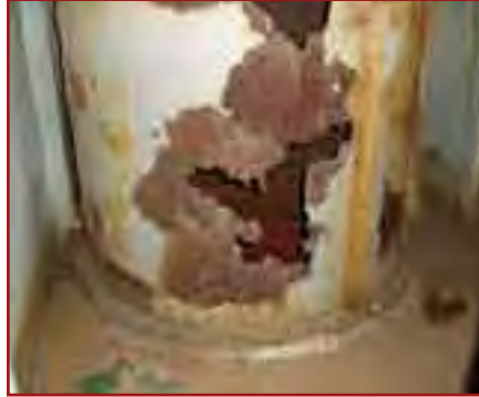
Engine room fire dampers
