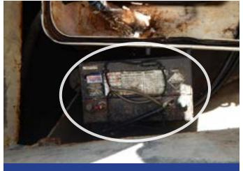
This battery is not contained within a battery box or adequately secured. Wing nuts are not considered adequate terminations for battery connection.
