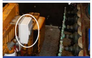
This sub board is unsuitable for its location. There is no cover on the circuit breakers, exposing them to the environment within the engine room, such as people walking past and possible leaks from the manifold directly opposite it.
