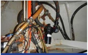
This photo shows untidy, bare conductor terminals. All connections need to be contained within junction boxes.
