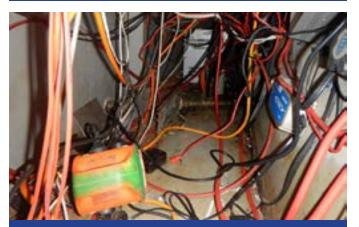
This photo shows unlabelled, unsecured mixed voltage wiring (a mixture of extra low voltage [ELV] and low voltage [LV] wiring) in disarray. In the event of a fault needing investigation, the messy collection of wiring would expose the person carrying out the inspection to the risk of electrocution. Any redundant wiring should be removed to make it easier to find a fault and the remaining wiring needs to be tidied up.
