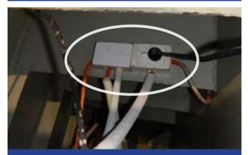
Cable entries need to be completed correctly, and conduits need to be supported to prevent stress on the wiring.
