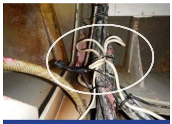
A junction box is required and the wiring needs to be tidied up and secured correctly.
