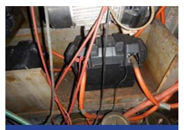
The battery box is not secure and allows possible venting of hydrogen gas to the ignition source on the water pump above.
