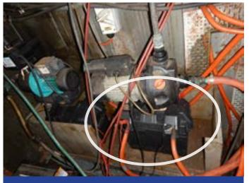
The battery is directly below a source of ignition.
