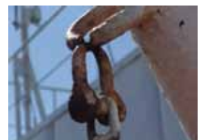
Damaged lifeboat davit
