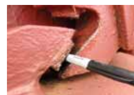
Hatch cover cleaning system - Excessive clearance
